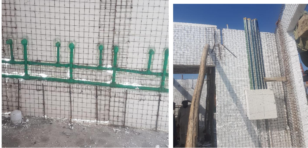
Figure 07: Installation of utilities before concretion
