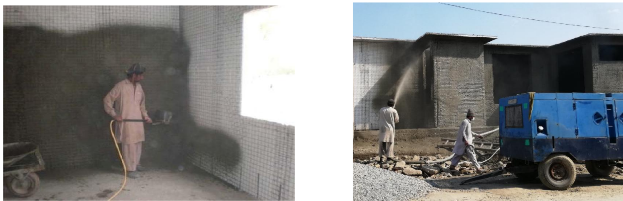
Figure 08:Applying Concrete
