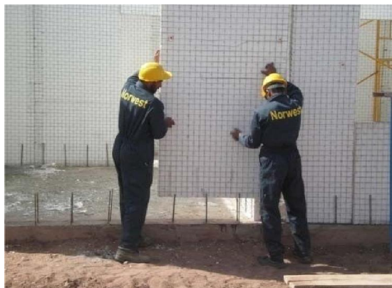
Figure 05 : Placing panels in dowels
